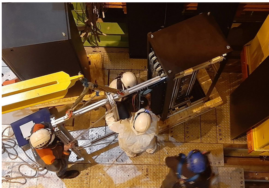
Transfer from the Cabinet to the Handling Frame
