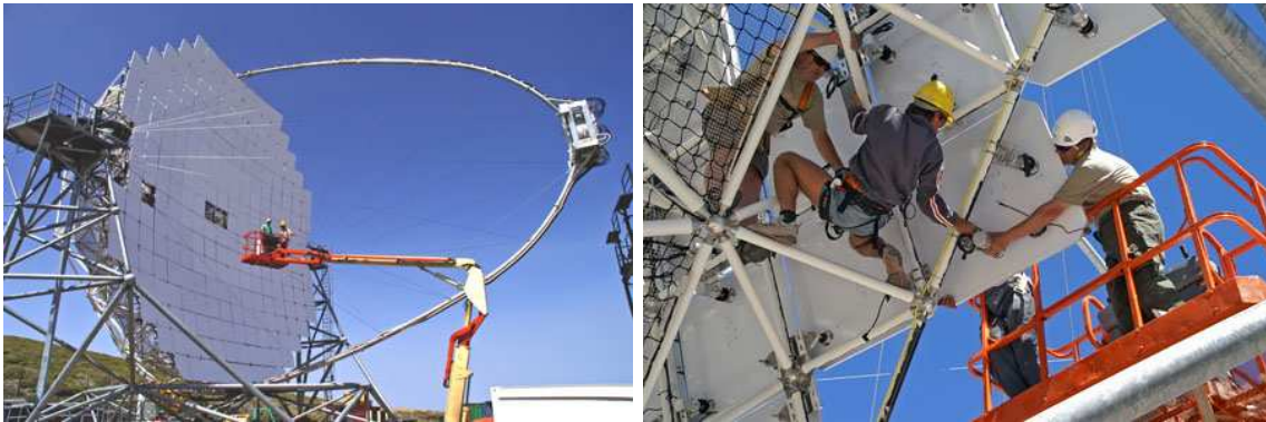
Figure 4.34: Two phases of the installation of the mirrors in the telescope. The mirror is taken to the reflector front via a cherry-picker (left) and the mirror is fixed by operators to pads mounted on the telescope structure.
